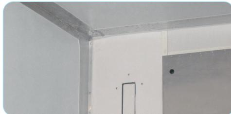
Less fasteners and Utility's FDA compliant lining, mean less locations for moisture to get trapped. Moisture traps are where pathogens can grow. The extruded aluminum lining corner closures are engineered with capture channels that don't require fasteners. The Utility design ensures best in class cleanability using industry standard practices, helping you achieve FSMA compliance.
